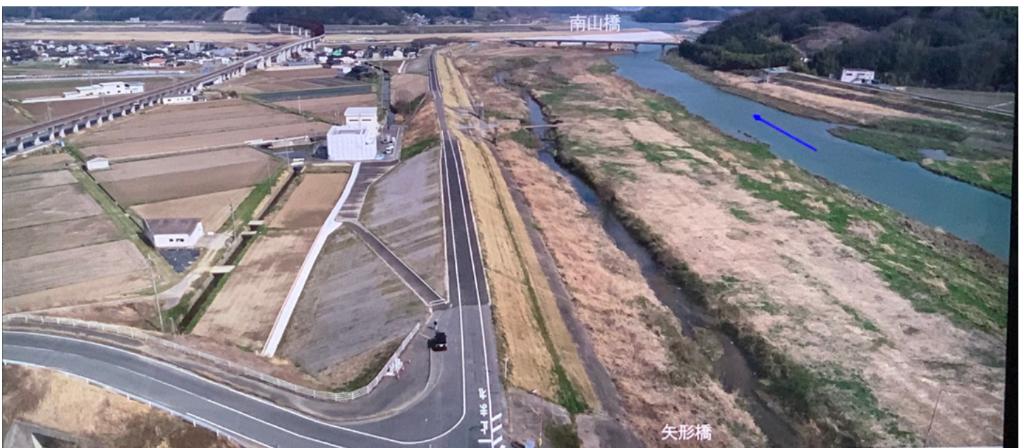
PICTURE 3: Levees along Oda River after completion (source: MLIT Mabi Bureau)
