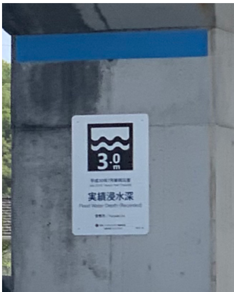
PICTURE 6: Example of blue line (showing the height of water during the 2018 flood)
