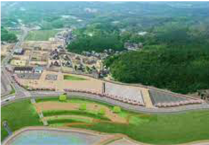
PICTURE 5: Image of the River Disaster Prevention Station (Source: Document published by MLIT Chugoku Regional Bureau)
